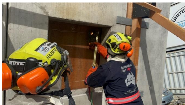
Figure 2 USAR operations hot cut to access a casualty.
